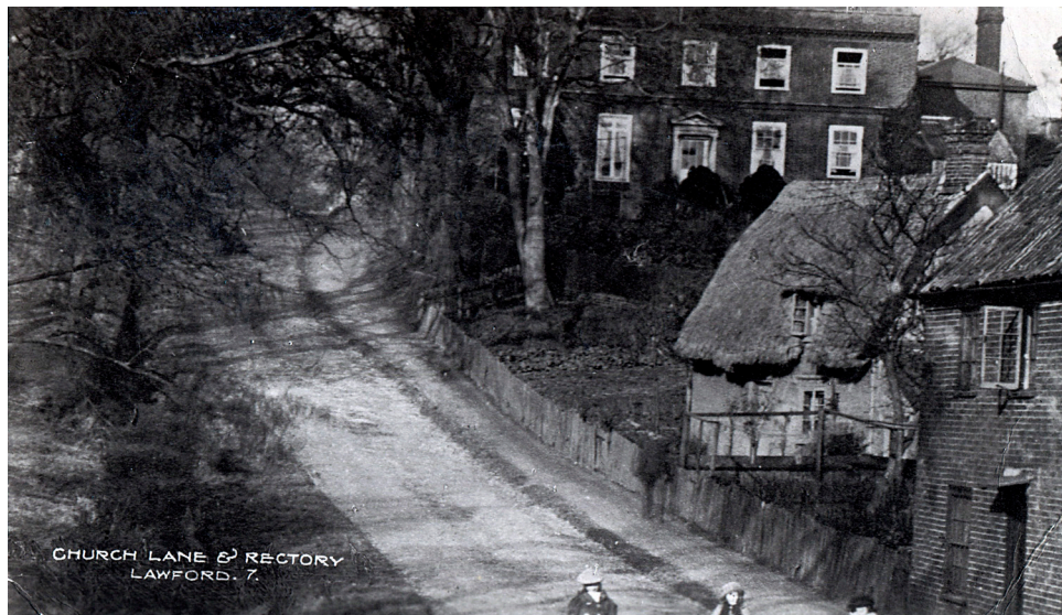
Figure 5 Photo of Church Lane, Rectory
