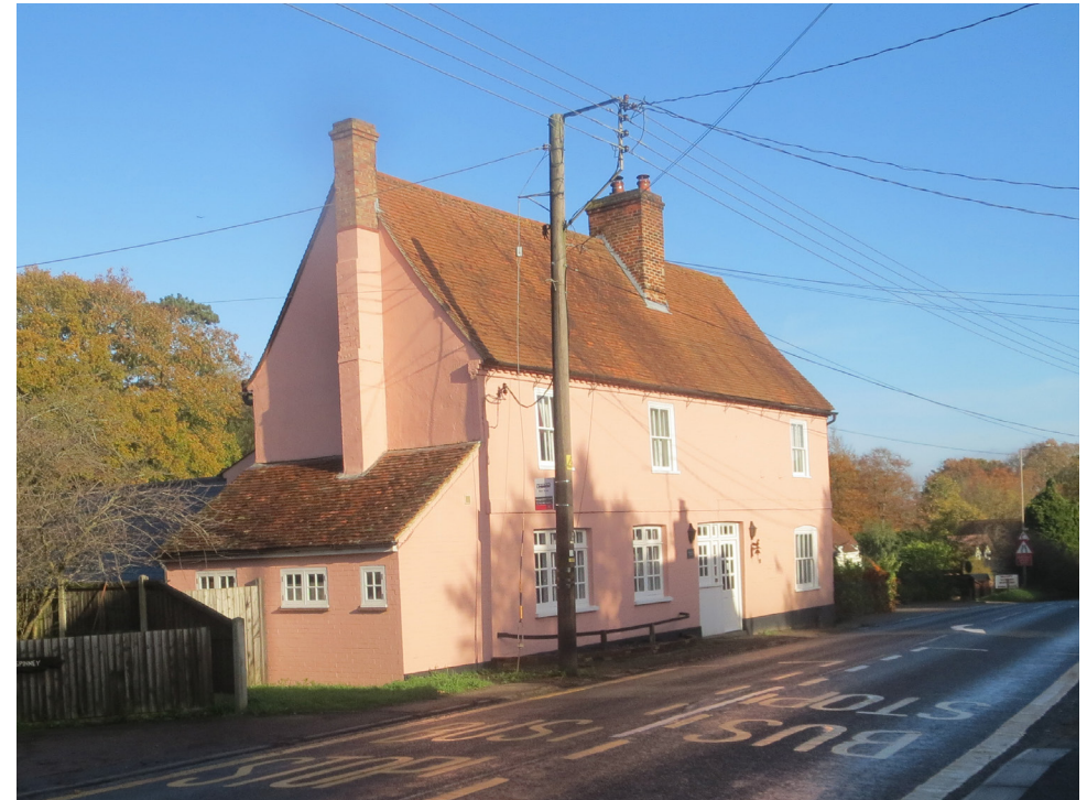
Figure 14 Photo of Kings Arms
